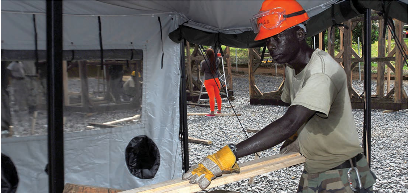
A Liberian military engineer cuts wood braces for the Tubmanburg Ebola treatment unit. In 2014, DLA Troop Support Construction and Equipment's maintenance, repair and operations program supported Operation United Assistance, the Defense Department's operation to help contain the Ebola virus in West Africa.
